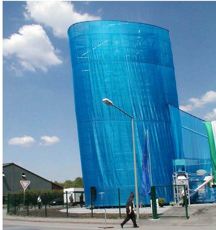
Pilot plant “Blauer Turm” in Herten, North-Rhine-Westphalia, Germany
